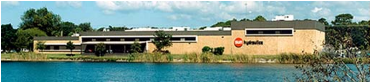
Sun Hydraulics Corporation, Sarasota, Florida
